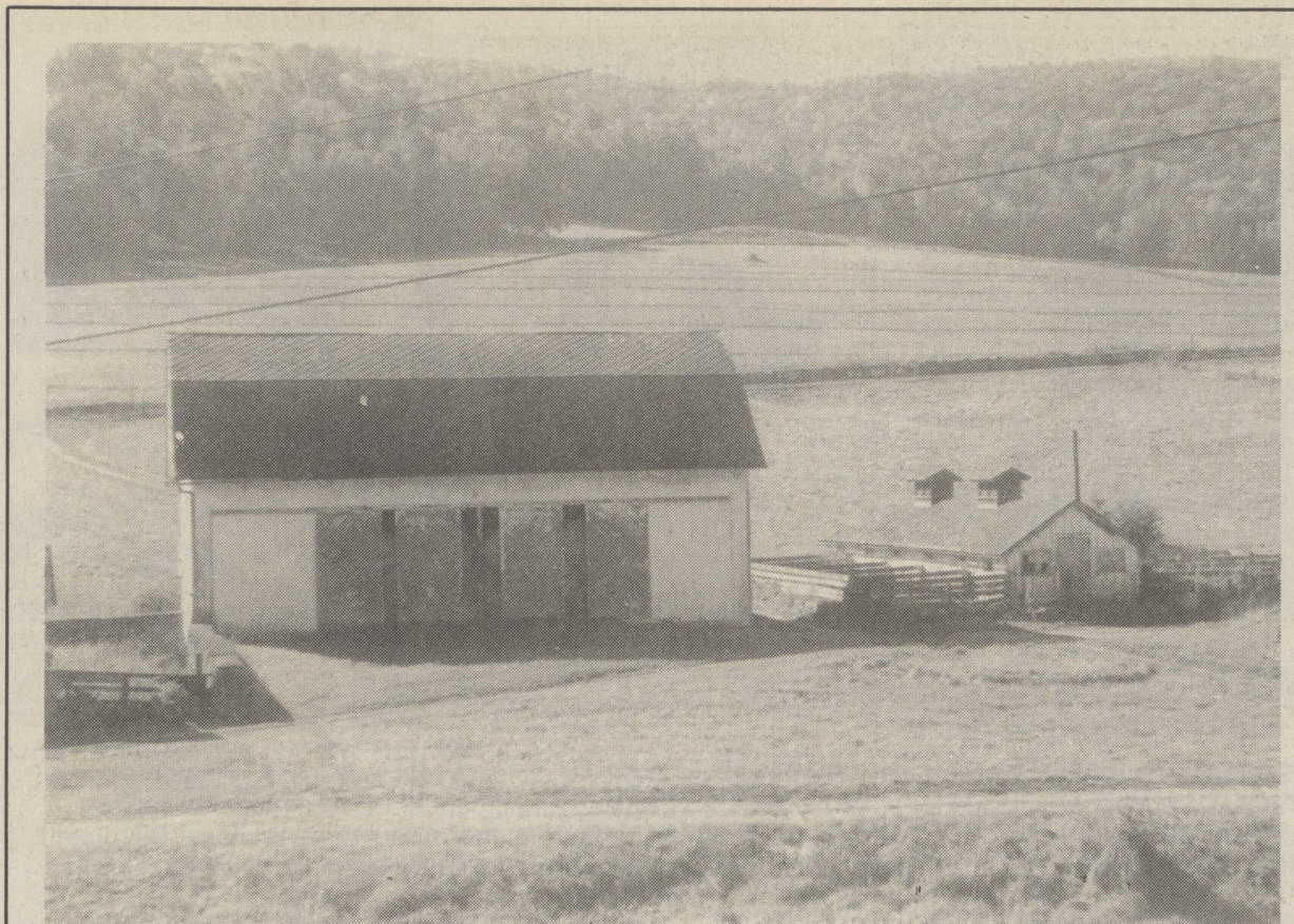
Barn from Hillside Road, Trucksville. Photo by Charlotte Bartizek.
