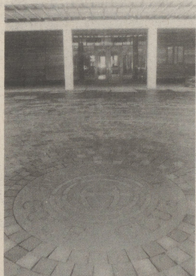
POST PHOTO/CHARLOTTE BARTIZEK Paving blocks of Pennsylvania bluestone form a large plaza at the entrance of the clubhouse, with the club's name inscribed in a large circular stone. Imposing Mahogany benches flank the entrance doors.
