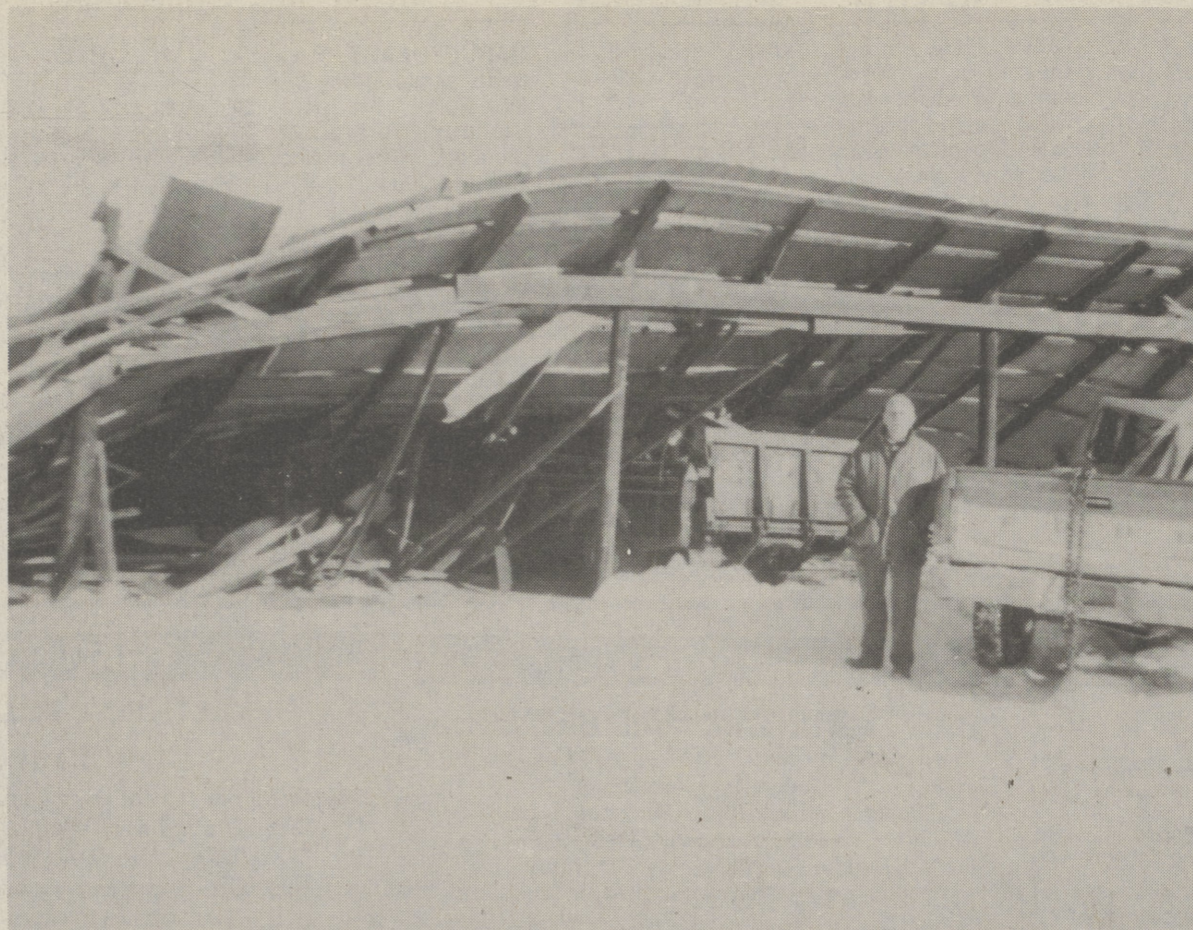
IT WASN'T AN EARTHQUAKE - Alan S. Major surveys two Ford pickup trucks crushed when his pole barn in Lehman Township collapsed from the weight of the snow January 19.
