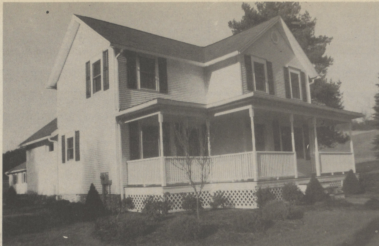
ALL FIXED UP - The old tenant house on the former Schooley Farm in Shavertown gained new life when renovated by the Burak family. (Post photo/Charlotte Bartizek)
