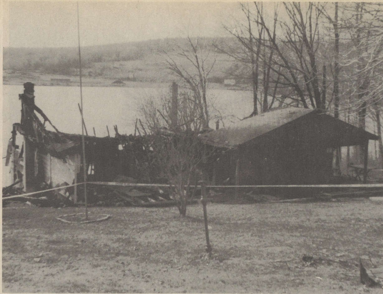
FIRE CLAIMS A LIFE - This ranch home on Perrin's Marsh, Franklin Twp., was destroyed in a fire which claimed the life of Ella Mae Christian early Saturday morning, April 11. Firefighters from six area fire companies battled the blaze. (Post photo/Grace R. Dove)
