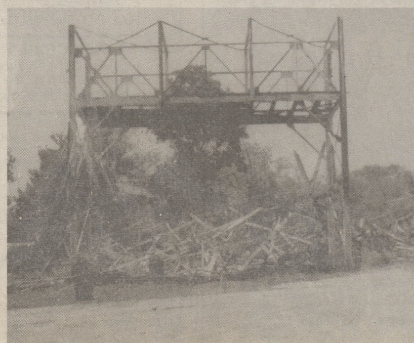
END OF AN ERA - This is all that remains of the wooden roller coaster at Hanson's Amusement Park at Harveys Lake. The coaster, which was an attraction at the park for nearly 50 years, was demolished July 10. Many residents have fond memories of the roller coaster and the amusement park, which has been closed since 1984. (Post Photo/Rich Johnson)
