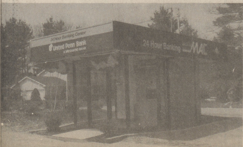
IN THE WRONG PLACE - This MAC machine in Dallas Twp. is installed where it may cause problems for an adjacent neighborhood, say residents there.
