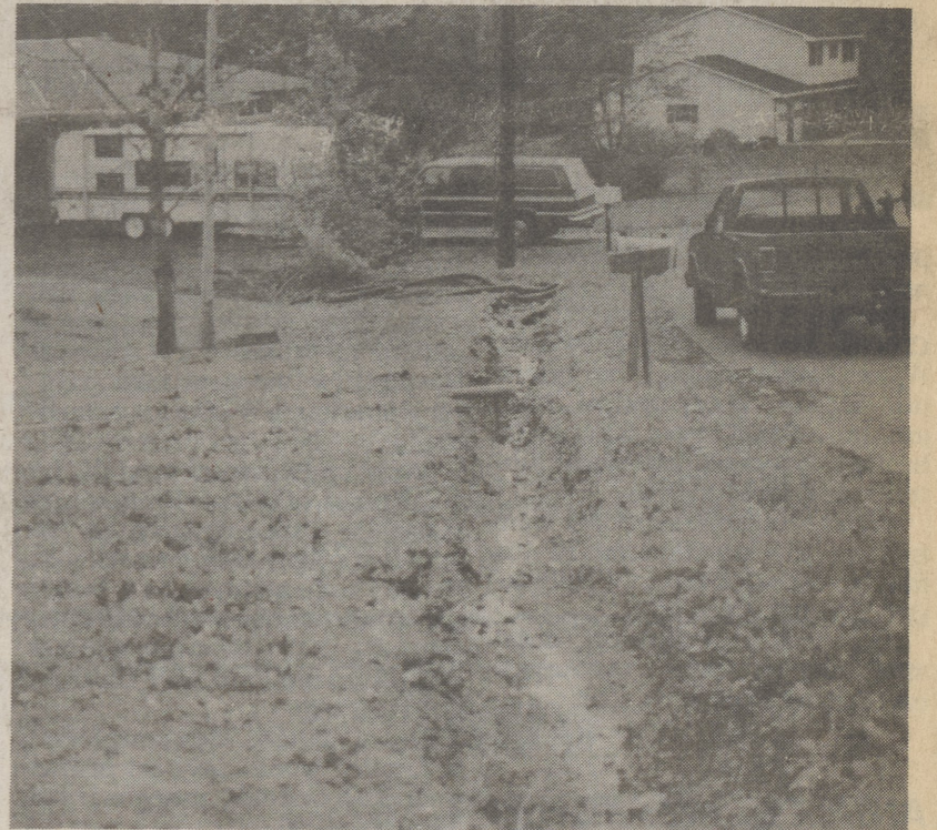
POOR DRAINAGE - This drainage ditch cuts through a driveway in Town & Country Manor in Lehman. Property owners are asking the township to correct runoff problems. (Photo contributed)
