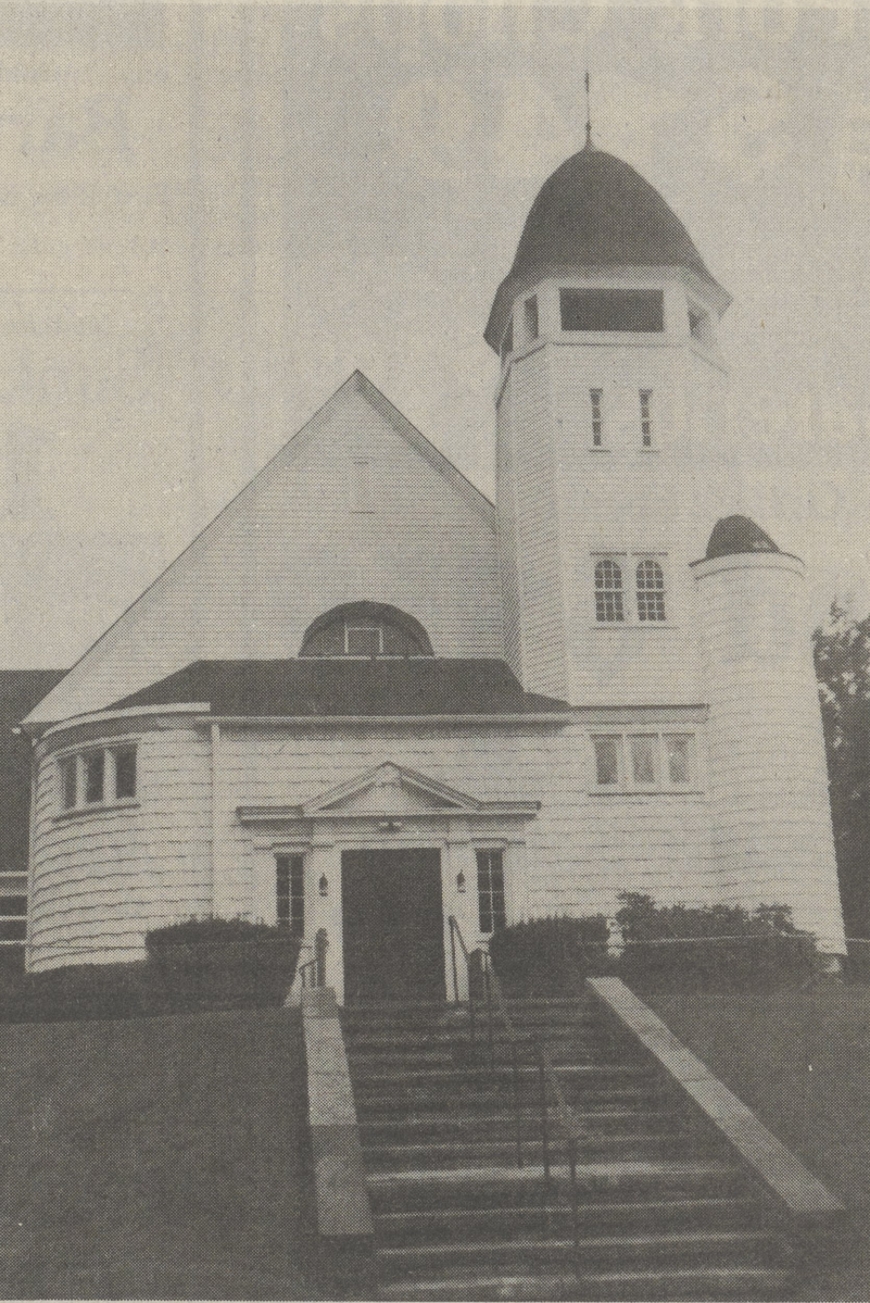
DUE FOR A SPRUCE-UP - The Dallas United Methodist Church will be receiving major renovations during this, its 100th year. (Photo by Charlotte Bartizek)
