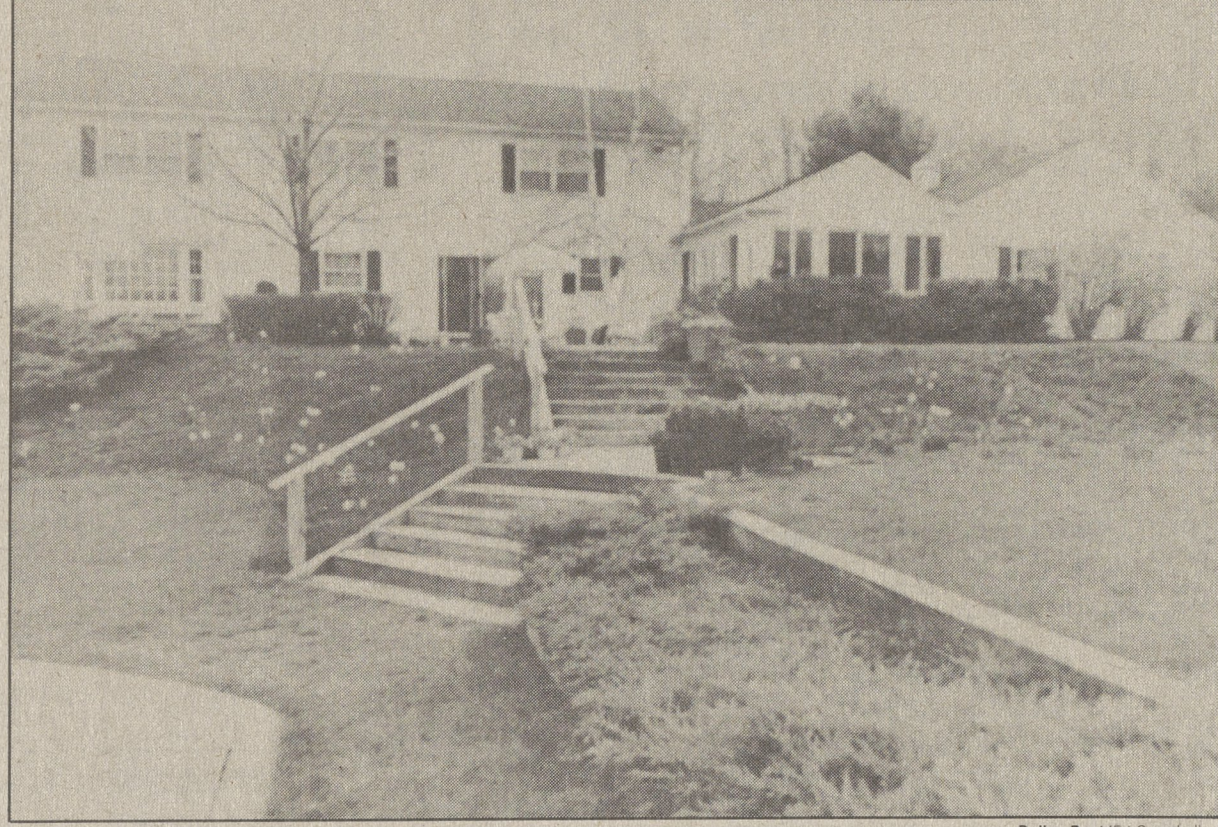
Rear view of Decorators' Show House
