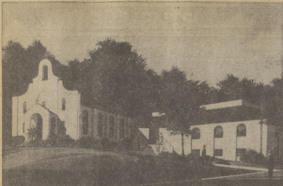
CHURCH RENOVATIONS - Our Lady of Victory Church, Harveys Lake, shown above, will soon have a new parish community center.
