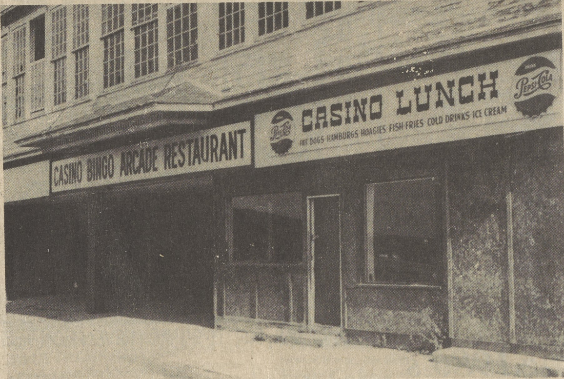
CASINO RAZED --The Casino at Harvey's Lake at one time was the entertainment center for the Sunset area. Bingo games were held downstairs while dances were going on up stairs. Various restaurants came and went in the front portion of the building along with game rooms. But with time comes age and the building has become an eye sore which will be torn down.
