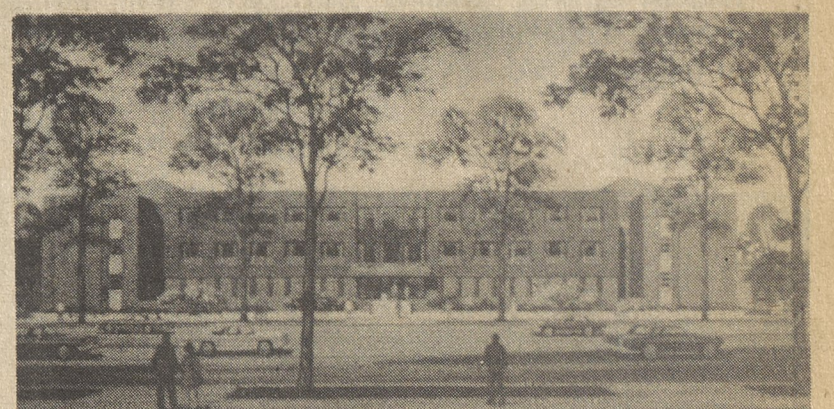
HOSPITAL--Artist's painting of Nesbitt Memorial Hospital which will complete its building program in 1983.
