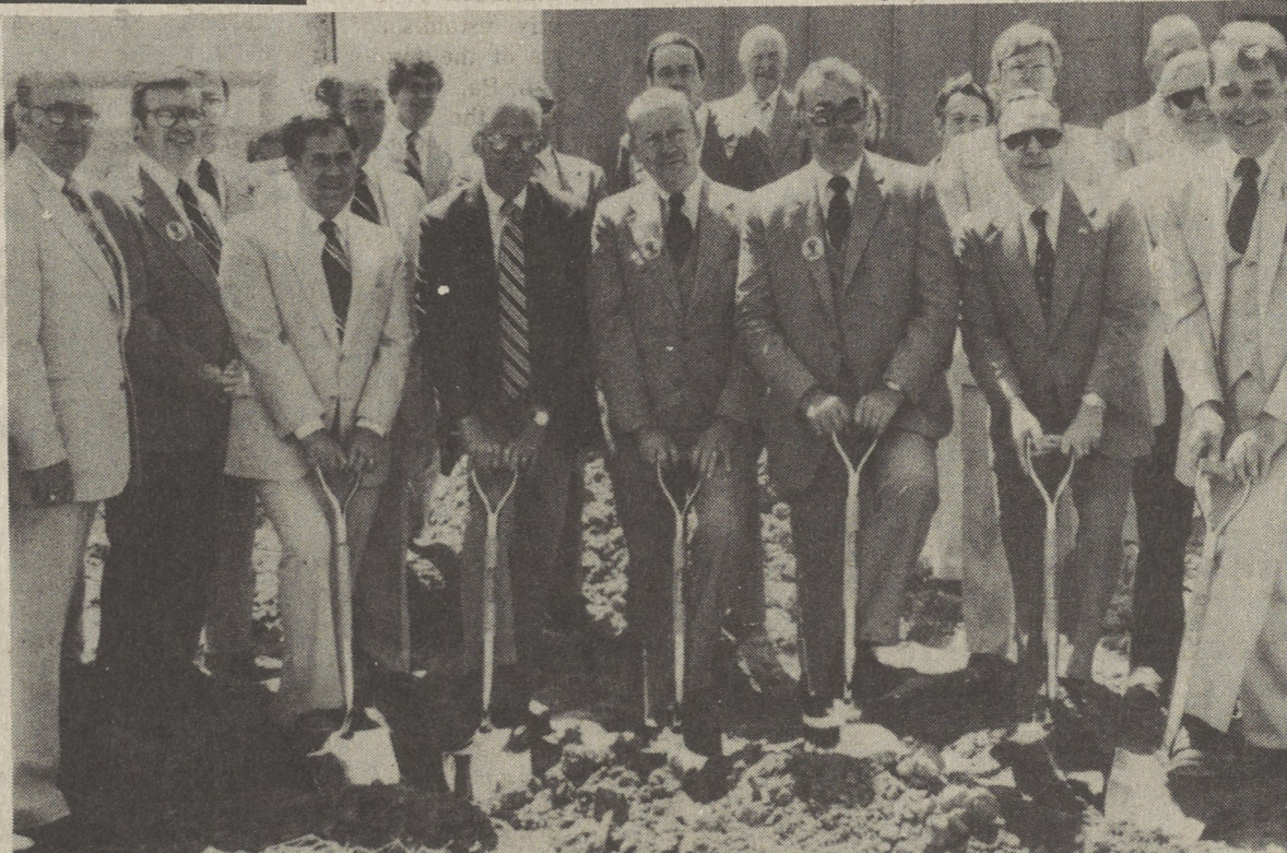
BANK GROUND BREAKING —Northeastern Bank officials at the groundbreaking for the bank's Back Mountain Branch are shown as they turned over the ground at the building site on Route 309. Left to right, with shovels, are Glenn Howell, manager of Dallas office; William Lees, executive vice president and chief
