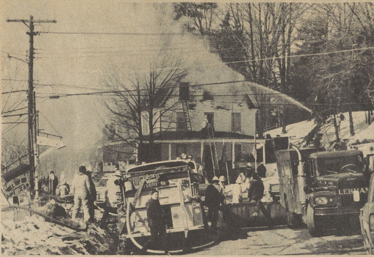
JUST THE BEGINNING - This is just the beginning of the damage done by the fire to Lakeside Hotel last week at Harveys Lake. The flames destroyed Tattersall's property and left more than 20 persons homeless.
