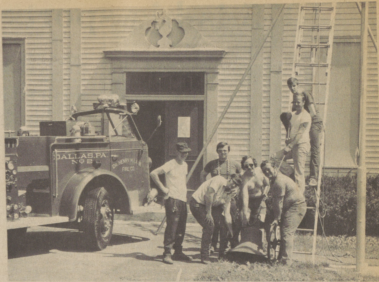
SCHOOL BELL—Members of the 1975 auction committee are shown above taking down the big bell from the top of Shavertown Elementary School. The bell was purchased at the auction by several dedicated volunteers and donated to the Back Mountain Library for use on the auction grounds.
