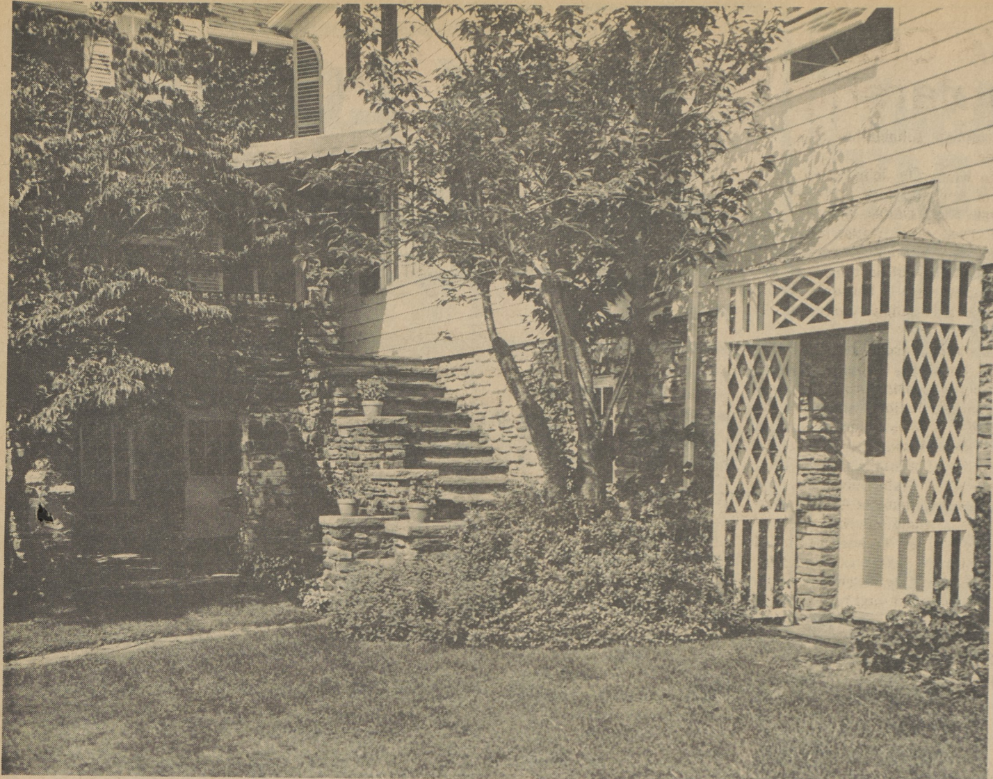
Pictured above is the home of Mr. and Mrs. John Troup, Shrineview, Dallas, which was built around 1930 by Pethick. The architect was Donald F. Innes. Points of interest here are the beautiful terraced grounds and the stone work shown in the picture which forms steps and a porch. The home also includes a sunken living room, many antiques and oriental rugs.
