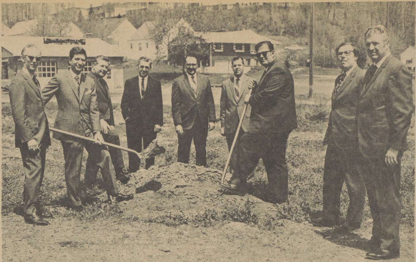
Shown breaking ground Friday for the new Weis Market in Dallas on land between Routes 415 and 309 are Robert Weiss, with shovel at left, and Steven Hartman, right. Looking on are, left to right: Paul Rodda, Joseph S. Yuschock, Thomas H. Kiley, John C. Coleman, Robert Richardson, Henry V. Null and Herbert J. Morris.
