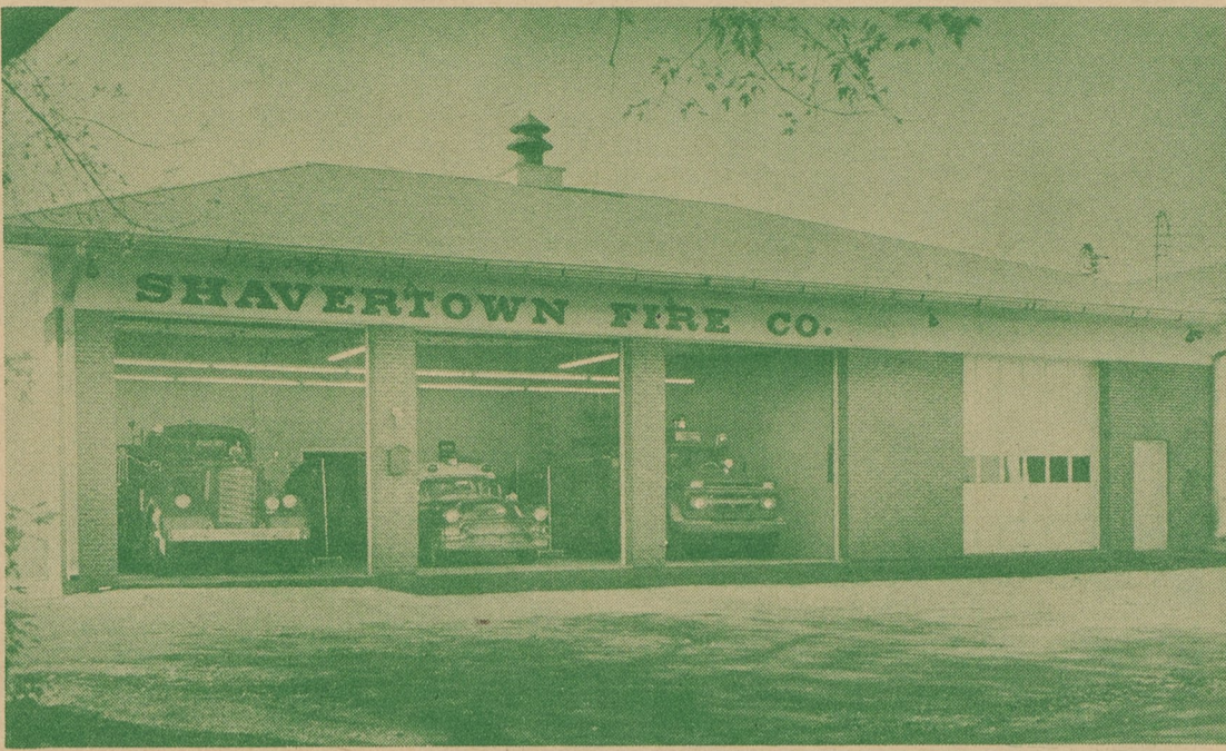
Community buildings also benefit from modern electric heat. Shavertown Fire Company is an excellent example of the latest developments in modern electric heating.
