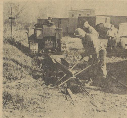
The wreckers are seen here pulling up rails and fastenings on the abandoned Lehigh Valley Railroad line from Luzerne to Noxen, expecting to finish some time in July. The contractor, Solomon Wrecking Company, Wilkes-Barre, says the sled being pulled behind the crawler tractor rips up rails in one day equal to what four men would do in a week.
