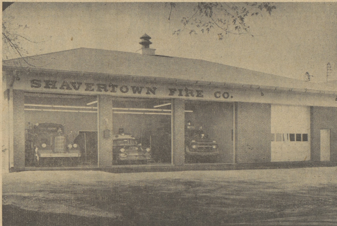
The Shavertown Fire Company proudly displays its new ultra modern Fire House which is totally heated and equipped with Care-Free Electricity.
