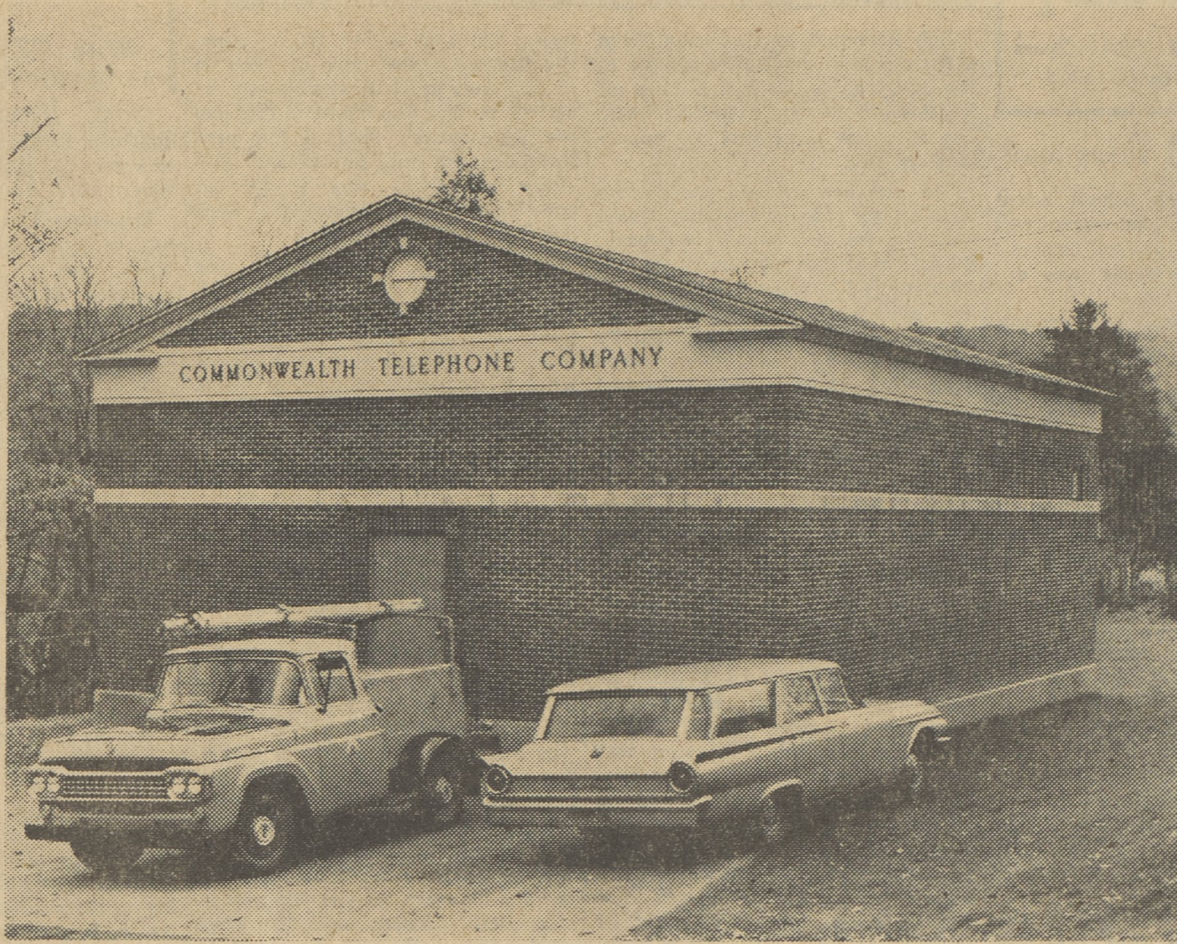
Top Center: Commonwealth's attractive new Dallas South exchange, 33' x 42', is located on Lewis Avenue, just off of Harris Hill Road. The attractive building, blends well into the contour of the land. A basement portion contains the cable vault into which the cables run, and a thermostatically controlled heating unit which maintains a constant temperature and humidity to protect the delicate dial switching equipment.
