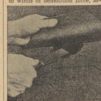
phalt shingle roofs can be made windtight by cementing down the shingle tabs. The cement holds the tabs down so that wind can-
