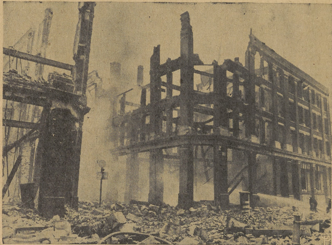
Gutted and reduced almost to rubble, these buildings were hit by German incendiary bombs during an air raid over London. Air raid precaution workers are shown extinguishing the last of the fire in the wrecked buildings.
