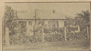
The new home of F. B. Moellers, where visiting poultry raisers are welcome.
