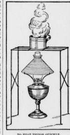
TO HEAT THINGS QUICKLY. permit of placing a lighted lamp un-demeath the top crossbars designed to serve as a support for the dish contain-ing whatever is to be heated. Braces on the sides prevent any collapse of the frame. The quantity of wire required is small and inexpensive, and the work of making the frame can be done in a comparatively short time with a pair of nippers.—Ladies' Home Journal.
