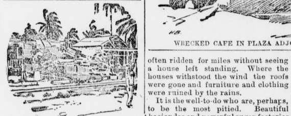
HOUSE IN PONCE DEMOLISHED BY THE HURRICANE.
