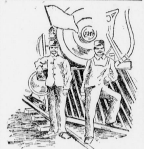
ENGINEER FITZGERALD AND FIREMAN.
