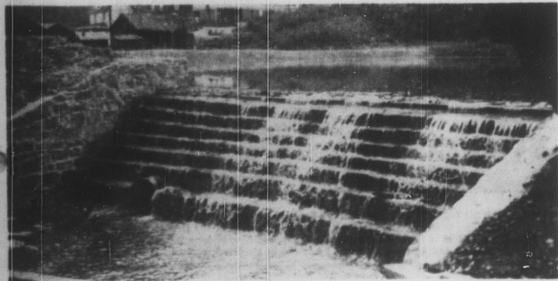
The spillway of the new dam is an excellent example of what can be done when a group of civic-minded citizens and sportsmen work together to complete a project for the mutual benefit of both groups. The spillway of cut stone is a tribute to the craftsmanship of the men who worked on the project in their spare time. The dam is located in the middle of the community of Dysart.
