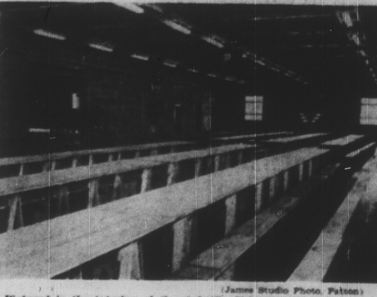
Pictured is the interior of the Ashville Volunteer Fire Company's new social hall, which was formally dedicated last month. The new hall which was constructed by volunteer labor from the town of Ashville, was built to replace an old building which was termed unsafe. Besides being used for weekly socials for the fire company, the new building is also used for roller skating and other community affairs.
