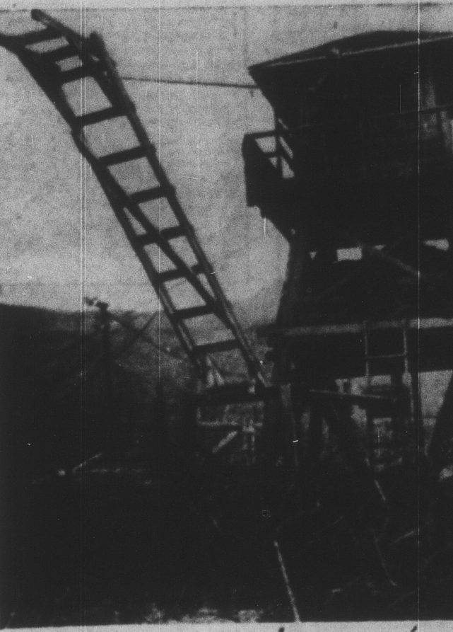
NECESSITY BEING the mother of invention, watchmen attached to this Koke Island prison camp guard tower rig up a device that defies the barbed wire entanglements of the compounds. It's a sort of drawbridge which can span the fences protecting the tower. (International)
