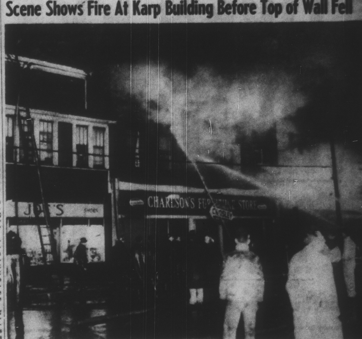
After ton of water was used in quelling the Thursday night and early Friday fire at Karp's building, volunteers from one of the companies called are shown here directing hose lines on the blaze.
