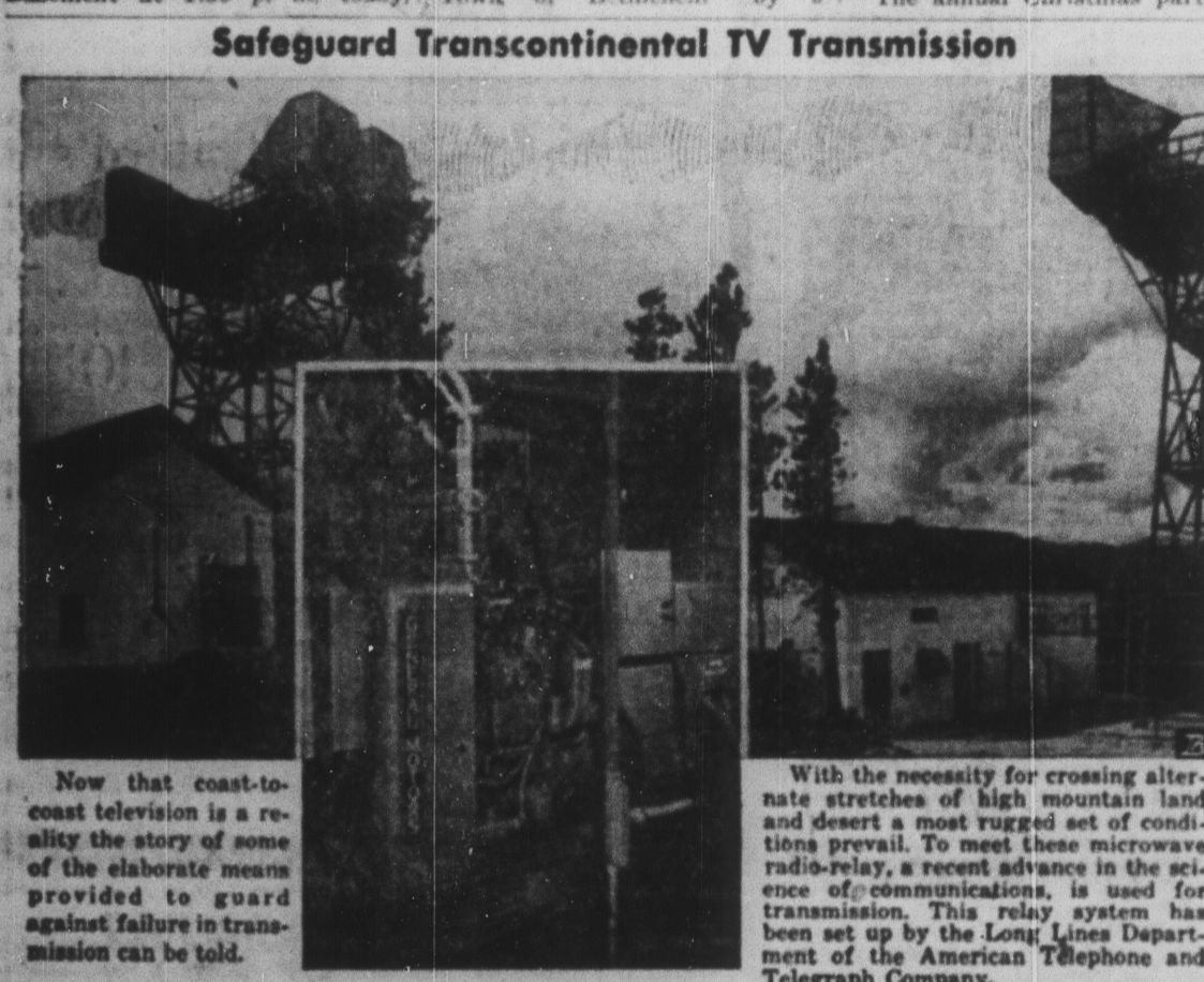
Now that coast-to-coast television is a reality the story of some of the elaborate means provided to guard against failure in transmission can be told. With the necessity for crossing alternate stretches of high mountain land and desert a most rugged set of conditions prevail. To meet these microwave radio-relay, a recent advance in the science of communications, is used for transmission. This relay system has been set up by the Long Lines Department of the American Telephone and Telegraph Company.
