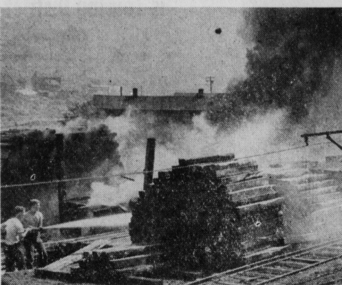
Parabaugh Studio Photo, Carrolltown Sterling Coal Co., Bakerton, suffered $500 damage Tuesday noon when a vat of creosote caught fire at its No. 6 mine tiple. Contents of the vat and a number of ties burned. Shown are Denny Weakland and Ed Bearer of the Carrolltown Fire Co. directing a hose on the flames. Dense quantities of smoke clouded the area.
