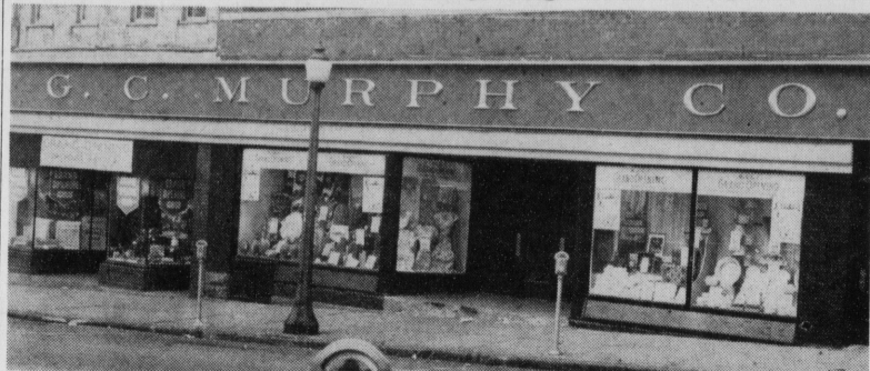
Pictured is the front of the new addition to the G. C. Murphy Co. store, Barnesboro, of which Harry Altman is manager.
