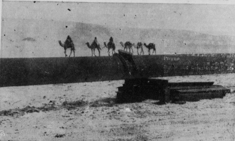
CROSSING VAST AREAS OF WASTELAND in Saudi Arabia, a camel caravan, ancient means of desert travel, passes the new 30-inch oil pipe-line now under construction there. When completed, the "Big Inch" pipeline is expected to send 450,000 barrels of oil daily from the Persian Gulf to the Mediterranean. (International)
