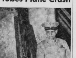
COMMANDING GENERAL of the Atlantic Overseas Air Technical Service Command, Brig. Gen. C. P. Kane inspects the scene of the disastrous bomber crash in New York's Empire State Building. He heads a four-man Army Board of Inquiry. Note part of the propeller shaft at lower left. (International)
