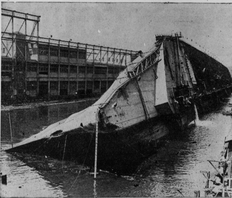
THE 79,280-TON HULK of the U.S.S. Lafayette (formerly the Normandie) is lifting itself slowly from the mud bottom of the Hudson River in New York, where it had lain on its side since it was swept by fire. Note that the superstructure had been cut away. The gauge at the prow gives the number of feet it has been elevated. The great liner is raising its hulk at the rate of a foot an hour. (International)
