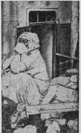
A STUNNED BERBER WOMAN sits amidst the ruins of her home in Casablanca which was blasted by German bombers on Dec. 1, 1942. Most of the damage was inflicted on the flimsy houses in the native section of the city.
