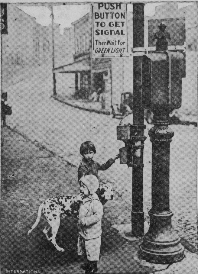
Pittsburgh has installed at busy traffic intersections a device by which the pedestrian can turn on the red light that stops vehicles and permits him to cross the street in safety. These little children are making use of it, the four-year-old boy pushing the button.
