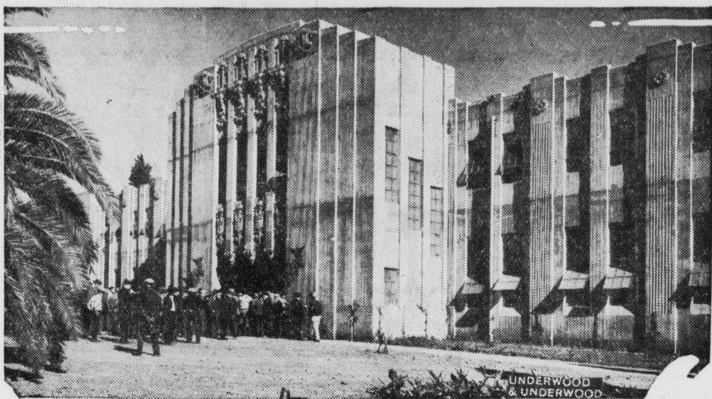
A striking view of the new modernistic mess hall at the National Military home at Sawtelle, Calif. This attractive building replaces an old frame structure which burned down, and is part of the program costing $1,000,000 of the $2,100,000 government appropriation for replacing old buildings with new brick, concrete and steel construction.
