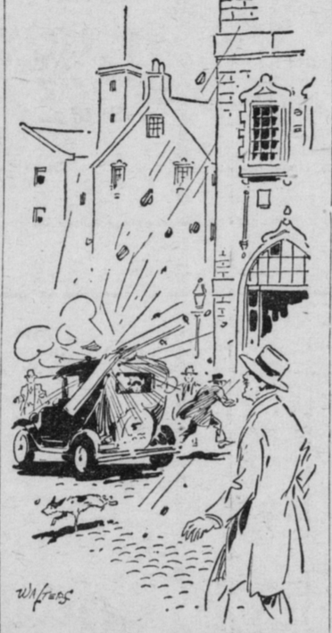
Afterward a Beam, Which Smashed a Motor Car.
