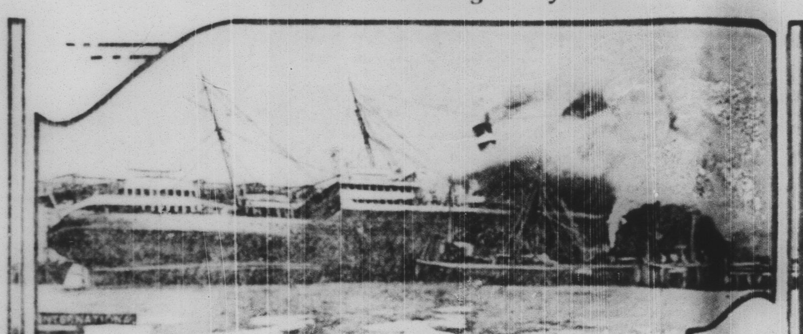
The S. S. America of the United States lines as she lay in her berth at Newport News where she destroyed almost the entire passenger quarters of the ship. The flames started, it is said from a blow torch. The ship had been at Newport News for some time being reconditioned, and was to have been turned over to her owners in a few days to resume her place in the United States lines service.
