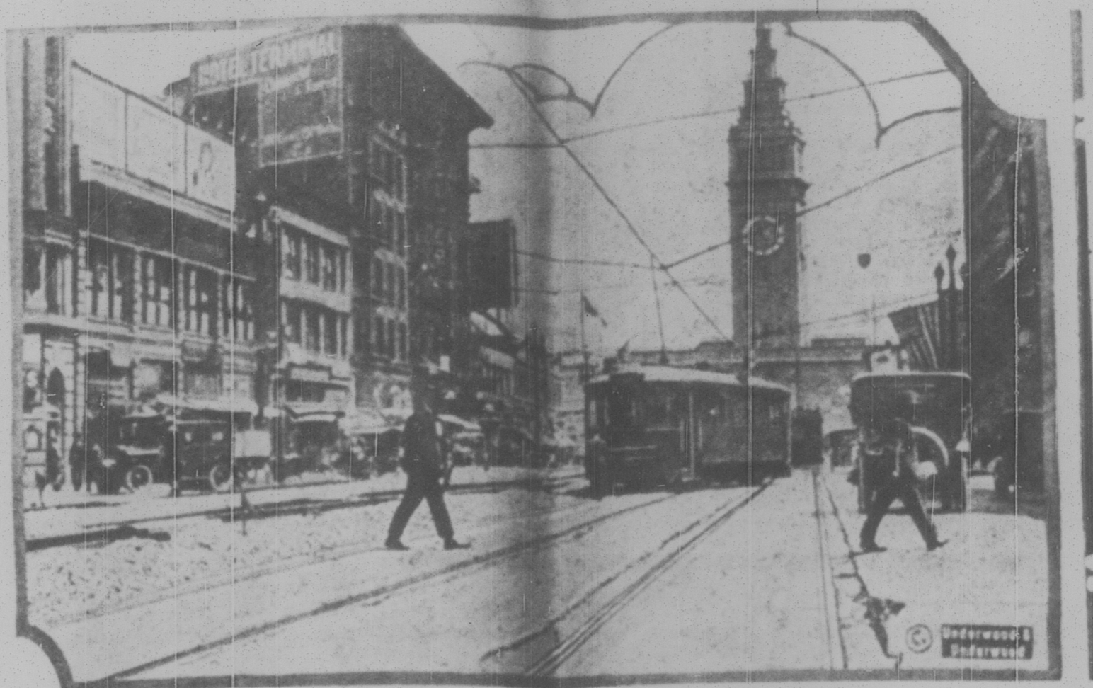
Weighted down by the tremendous tonnage of modern skyscrapers, Market street, San Francisco's main thoroughfare between the Ferry and First street, is slowly but surely sinking into the black mire of the bay. According to City Engineer M. M. O'Shaughnessy, the street has sunk 17 inches since 1906, or an inch a year. Steps will be taken at once by the city engineering department to prevent the encroachment of the sea.
