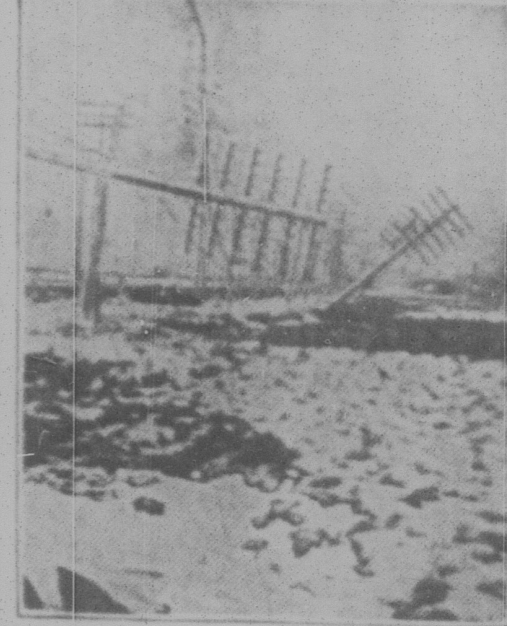
The tremendous burden of ice-coated telephone wires sometimes proves too great even for the strongest telephone poles.
