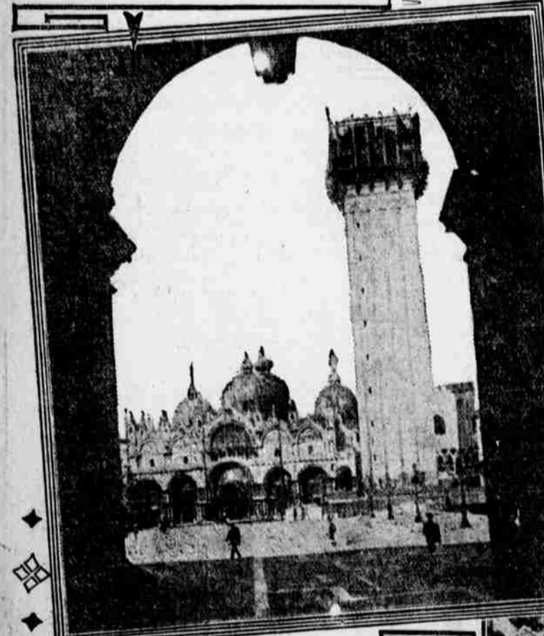
THE NEW CAMPANILE AS IT NOW IS
