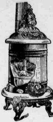
IN an ordinary soft coal stove, half of the coal arises in gas and promptly goes up the chimney. When you remember that gas is itself fine fuel, being used in all the large cities for cooking, heating and lighting, you realize how much is saved if the gas doesn't escape, but is held in the stove and burned.
