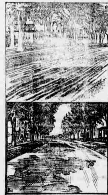
TWO PHOTOGRAPHS, SHOWING A ROAD BEFORE AND AFTER BEING DRAGGED.
