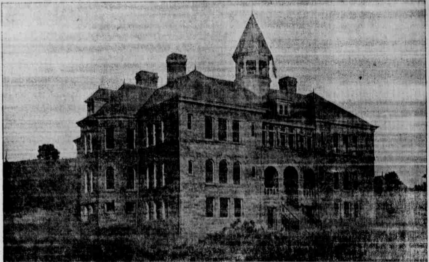
PUBLIC SCHOOL BUILDING—DESTROYED BY FIRE.
