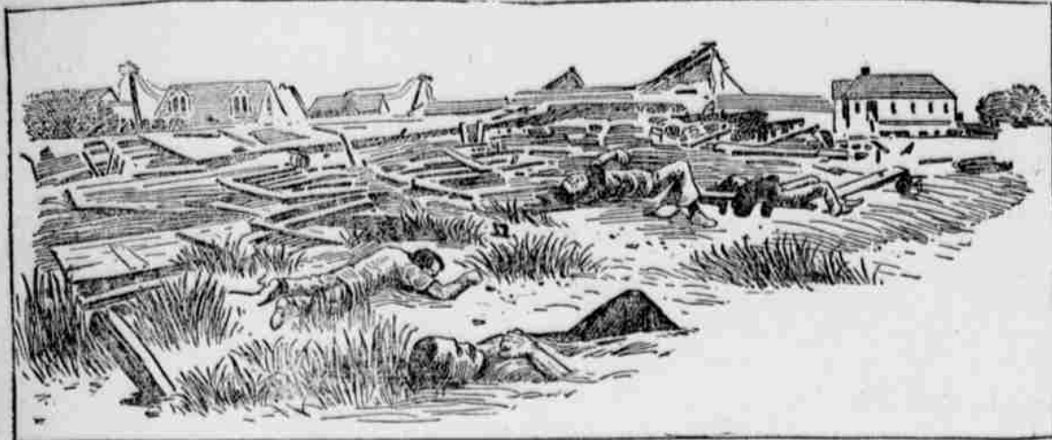
MORNING AFTER THE FLOOD NEAR BALL PARK, FOOT OF TREMONT STREET.
